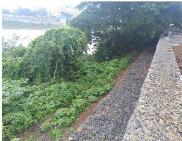
Top view of Gabion wall near water body
